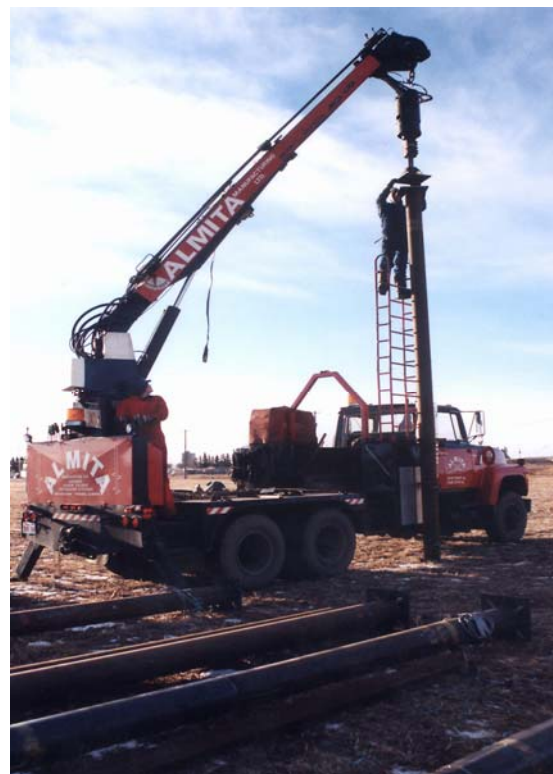
Figure 2. Screw Anchor Pile Installation
