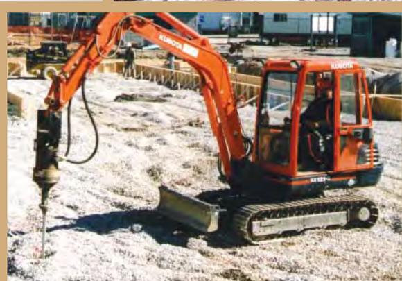
Installing helical foundations for structural slab support.
