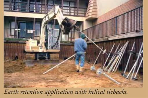
Earth retention application with helical tiebacks.
