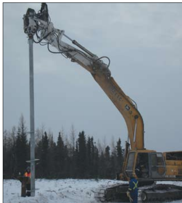
Figure 2. Typical pile installation
